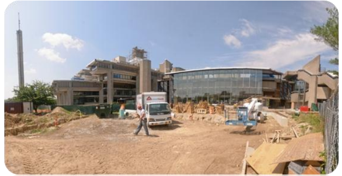
Figure 1 - Claire T. Carney Library & Curtain Wall Addition
